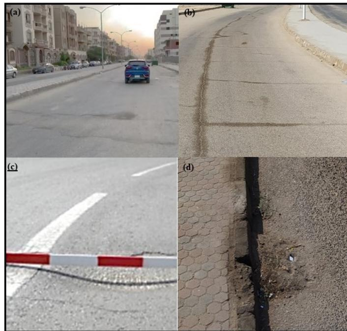
**Figure 4.** Typical distress patterns in the flexible pavement of the study network: (a) utility patching; (b) longitudinal and transverse cracking; (c) depression; (d) lane-to-shoulder drop off.
