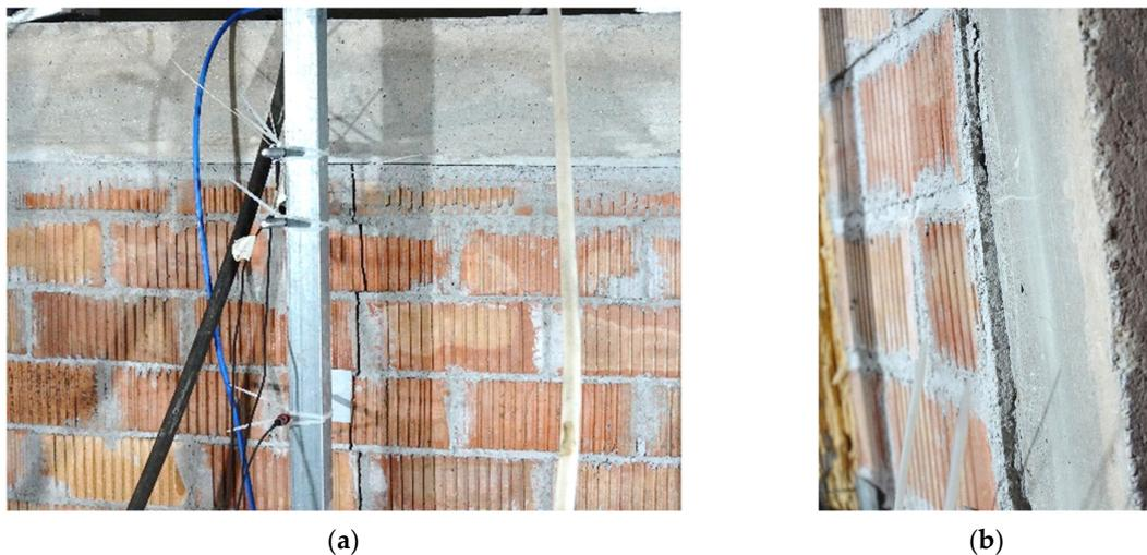
**Figure 19.** Infill wall damage: (a) vertical crack (URM wall); (b) detachment from lateral column (reinforced wall).
