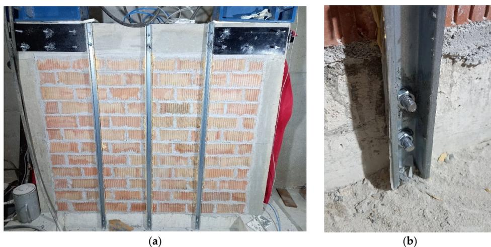
**Figure 16.** Reinforced infill wall: (a) overview of the infill wall reinforced by the structural renovation solution; (b) detail of the anchorage system between the omega profile and foundation.
