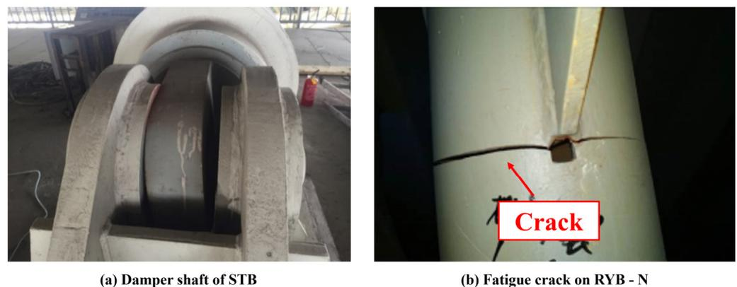
**Figure 7.** Local damage of the cable-supported bridges.
