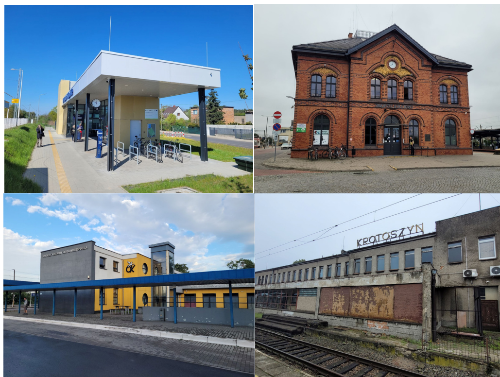
Figure 4. Different technical conditions and types of railway station buildings found in Poland in Biskupice, Jarocin, Środa Wielkopolska, Krotoszyn (own research work).
