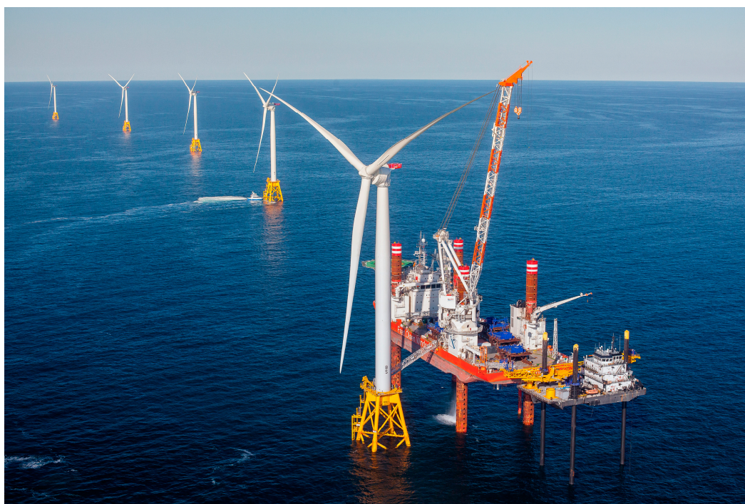
Figure 9. Installation of Turbines at the Block Island Wind Farm.
