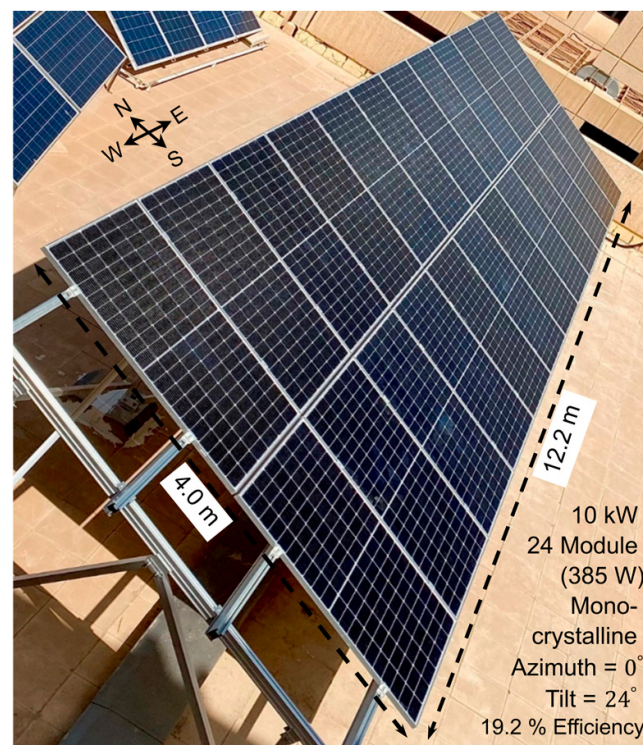
Figure 16. Laboratory-scale PV array used for case study analysis.
