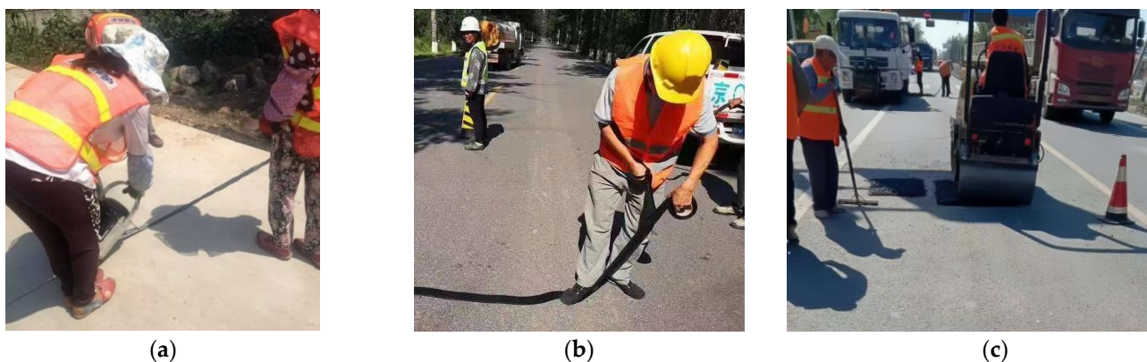
Figure 1. Traditional repair methods of crack and pothole: (a) pouring cracking, (b) sealing cracking, (c) digging-patching of potholes. (@Tai'an City Fang Shuo Engineering Materials Co., Ltd.).
