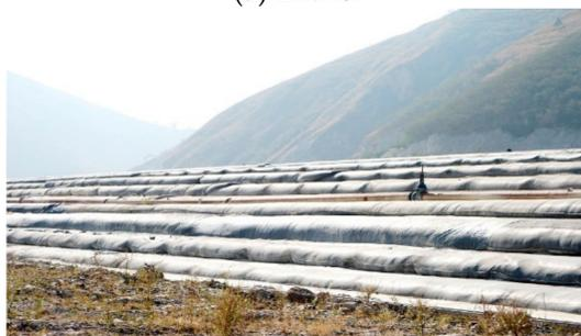
**(b)** Exterior**Figure 1.** Zoomed-in partial view of the tailings dam constructed with geotextile bags in Yunnan province: **(a)** interior; **(b)** exterior.
