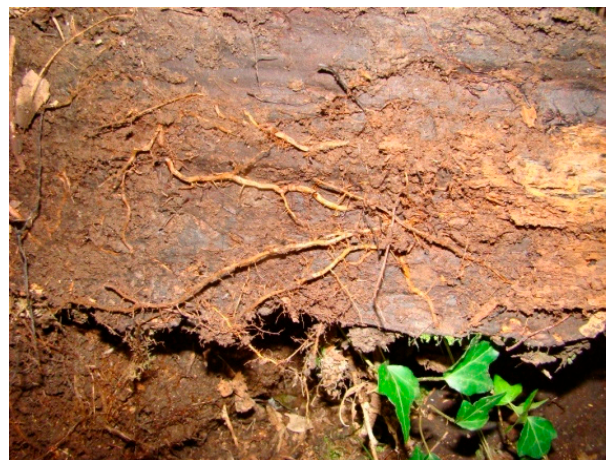
Figure 3. Crib wall logs in an advanced deterioration state (Artia river, Irún, Spain). Plant roots are occupying the space previously filled by tree logs while adsorbing nutrients coming from the decomposed wood. Source: Guillermo Tardio.
