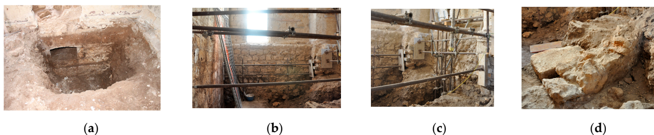
Figure 9. (a) The wall section (1) from the 16th century; (b) the wall section (2) from the 18th century; (c) the wall section (3), which possesses critical issues in respect of the foundations and (d) the wall section (4) that can be traced to medieval structures.
