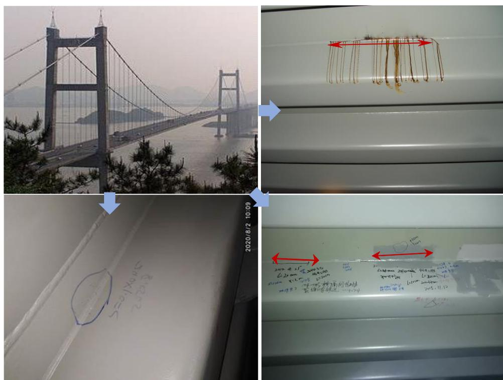
**Figure 1.** Typical fatigue cracks of Humen bridge.
