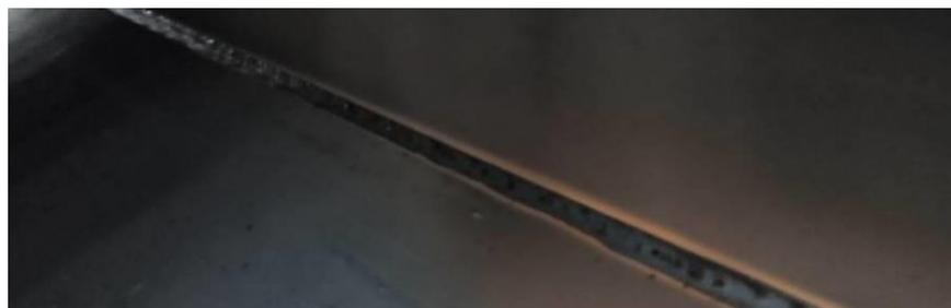
**Figure 3.** Weld seam at the inner side of rib-to-deck welded joints.
