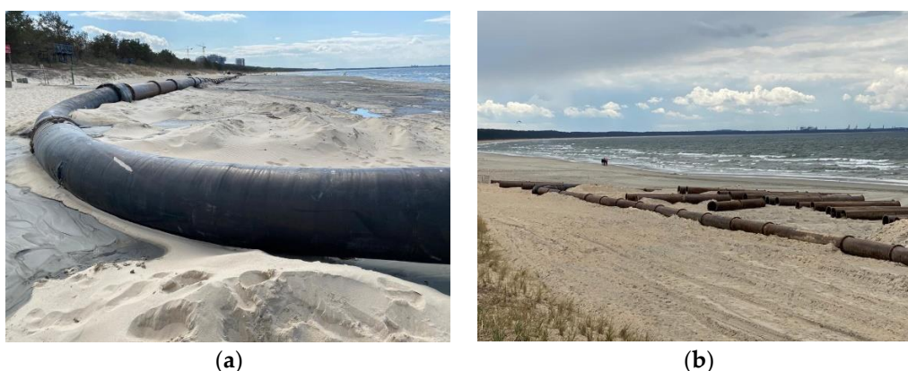
Figure 9. Counteracting the decline in the surface of the beaches as a result of the rising water level in the Baltic Sea. The technical process of increasing the level of the beach in Międzydroje using sand from the excavation for the deep-water Świnoujście gas terminal. Structure to strengthen and raise the level of the beach (a) main pipe transporting sand to the beach; (b) a piping system to transport the sand to the beach before installation. Photo by Z. Paszkowski.
