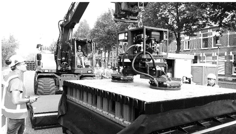
**Figure 2.** The currently available construction method of the prefabricated plastic panel for the cycle path (after [14]).
