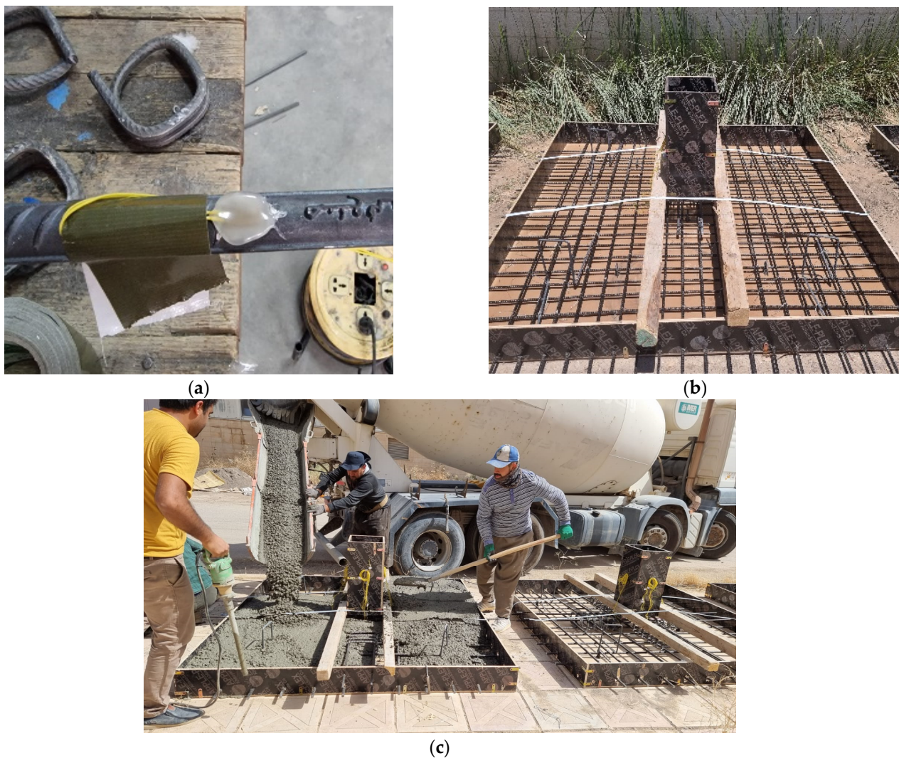
Figure 2. Construction of the samples: (a) strain gauge installation; (b) formwork and reinforcement placement; (c) concrete pouring.
