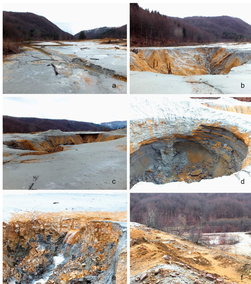
Figure 7. Târgu Lăpuș waste pond from Maramureș County (autumn 2016–2018): (a) surface water drainage; (b,c,e) suffusion processes in the extractive waste deposition area; (d) void created by internal collapse; (f) crest of the waste dump.
