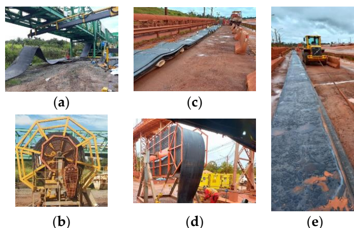
Figure 13. Pipe conveyor belt installation: (a) belt positioning; (b) belt winder; (c) folded belt; (d) flat round reel; (e) bulldozer pulling.
