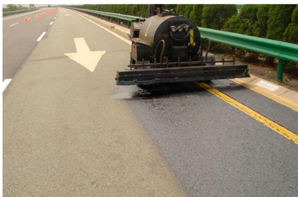
**Figure 2.** Fog seal technology with operation.
