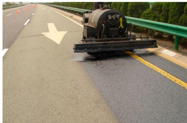
**Figure 2.** Fog seal technology with operation.
