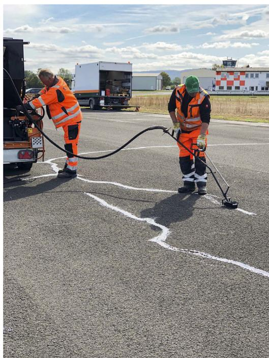
**Figure 1.** Hot pouring technology to heal the cracks.
