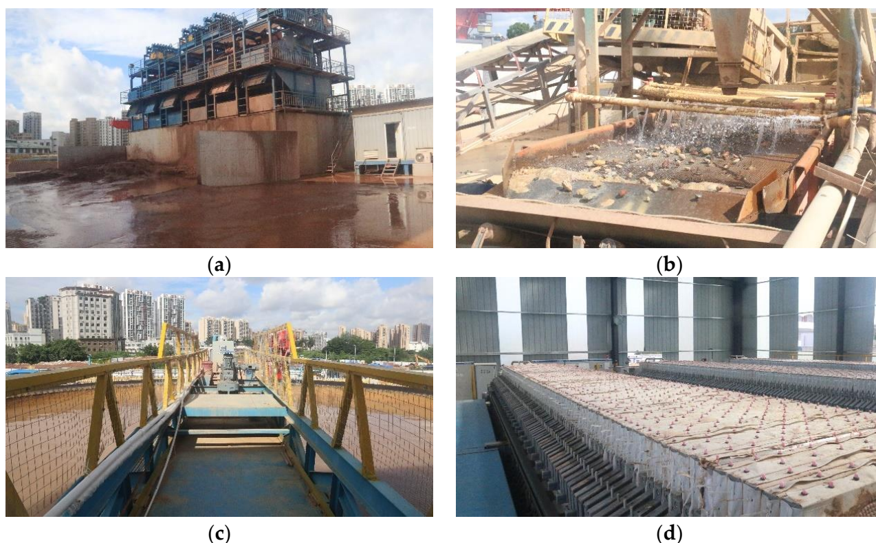
Figure 1. Shenzhen Metro Line 13 North Extension Project captured by on-site survey: (a) slurry separation; (b) mud swirling and screening; (c) flocculation–sedimentation; (d) filtration.
