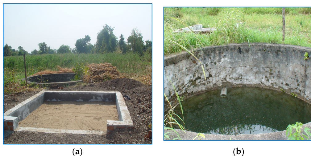
Figure 7. (a) Recharge filters attached with dug well, and (b) dug well at its full water storage capacity.
