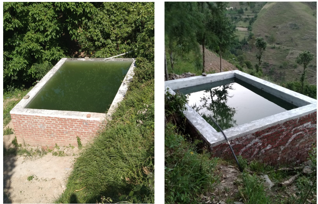
Figure 2. Spring-fed water storage tanks in Kumhali village of Shimla.
