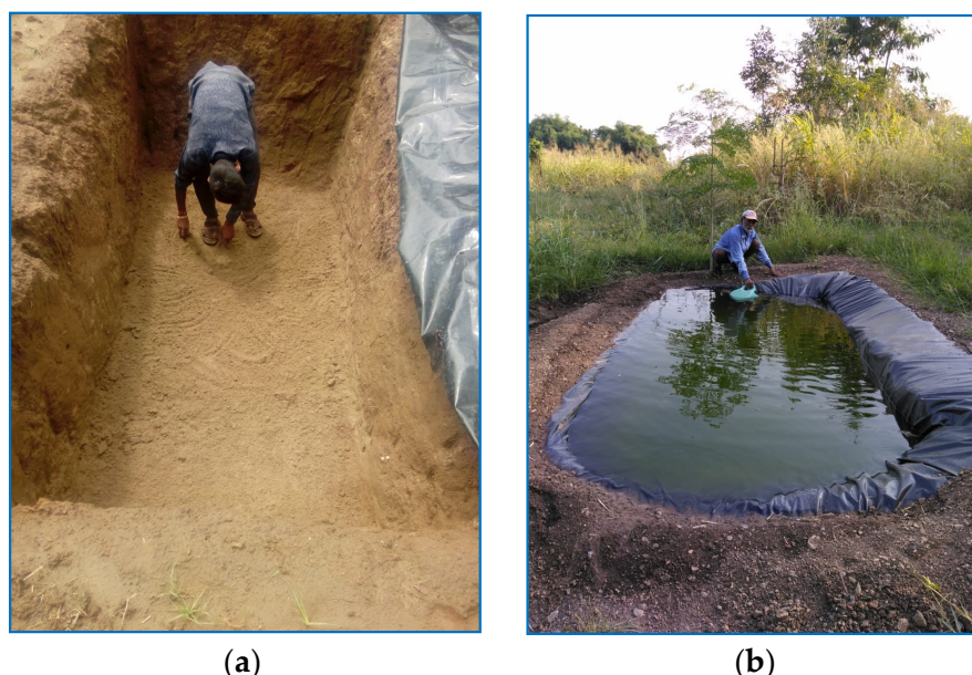
Figure 6. (a) Digging of pit in 2015 for construction of water harvesting pond (jalkund) and (b) plastic-lined pond.
