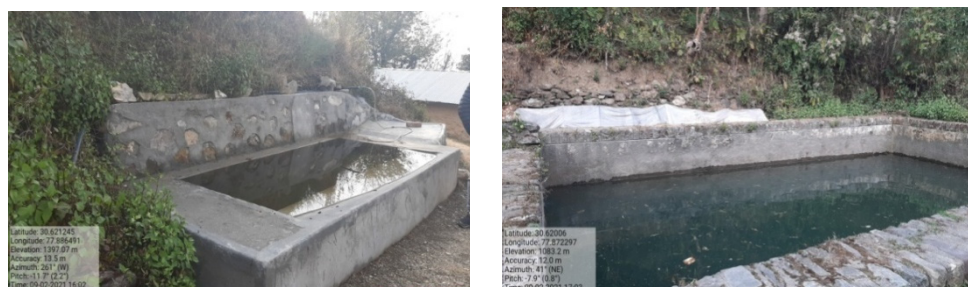
Figure 4. Spring water tapped, conveyed, and stored in water tank in Sahiya-Udpalta village of Dehradun.
