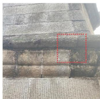
Cracks at the eave of the first floor
