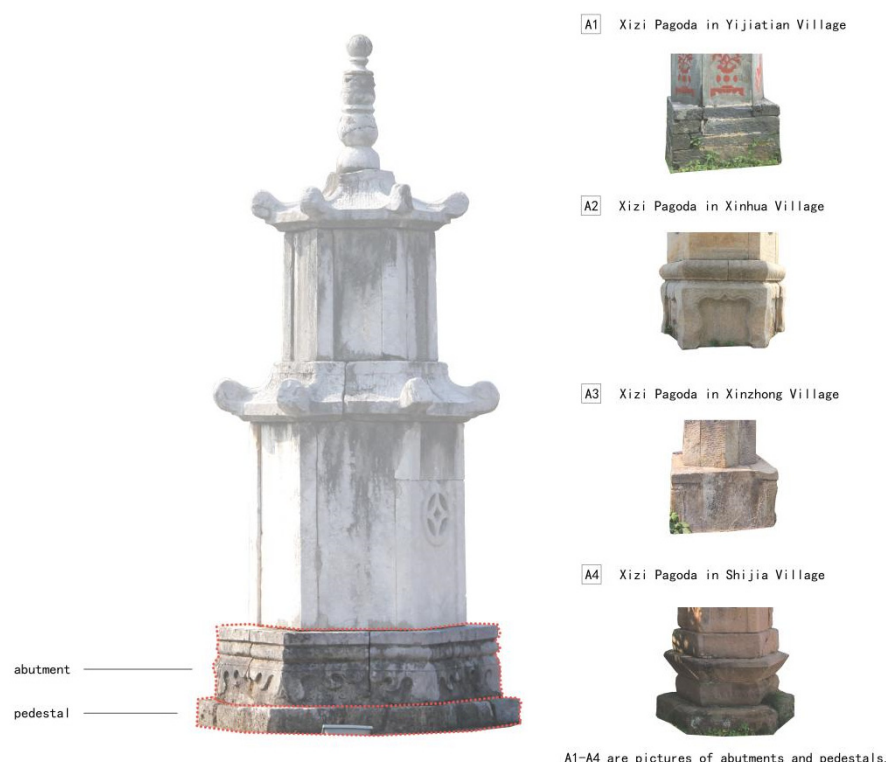
Figure 5. Foundation bed of the Xizi Pagoda (image source: made by the author).
