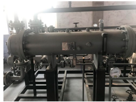
(b) Shell and tube condenser
