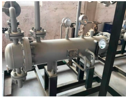
(a) Shell and tube evaporator
