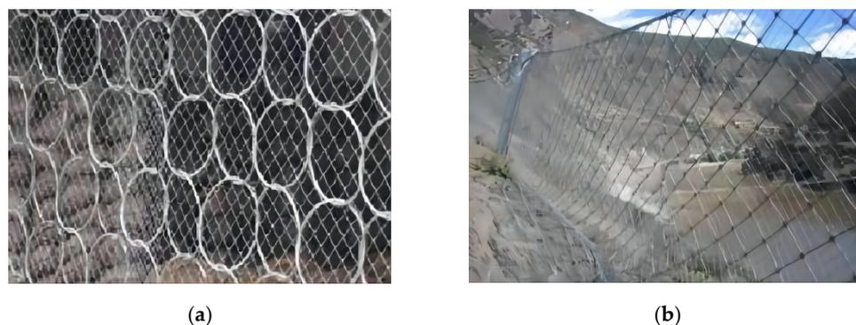
**Figure 3.** The form of passive flexible protective net. (a) Ring net; (b) Rhombic net.
