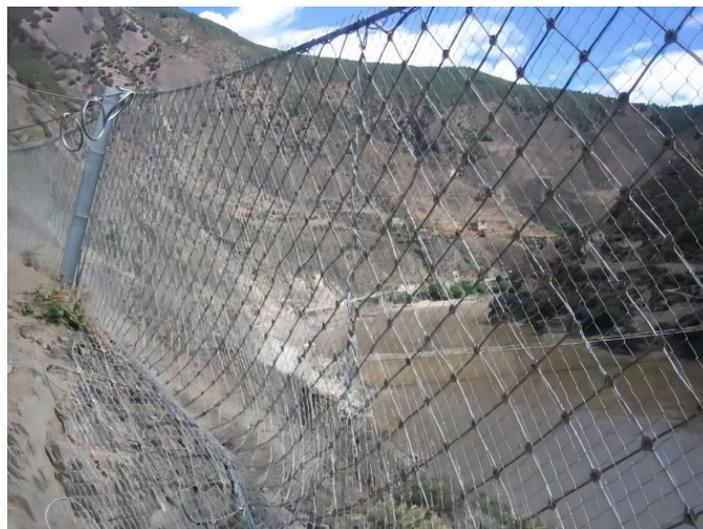
**Figure 2.** Application of passive flexible protective net structure.
