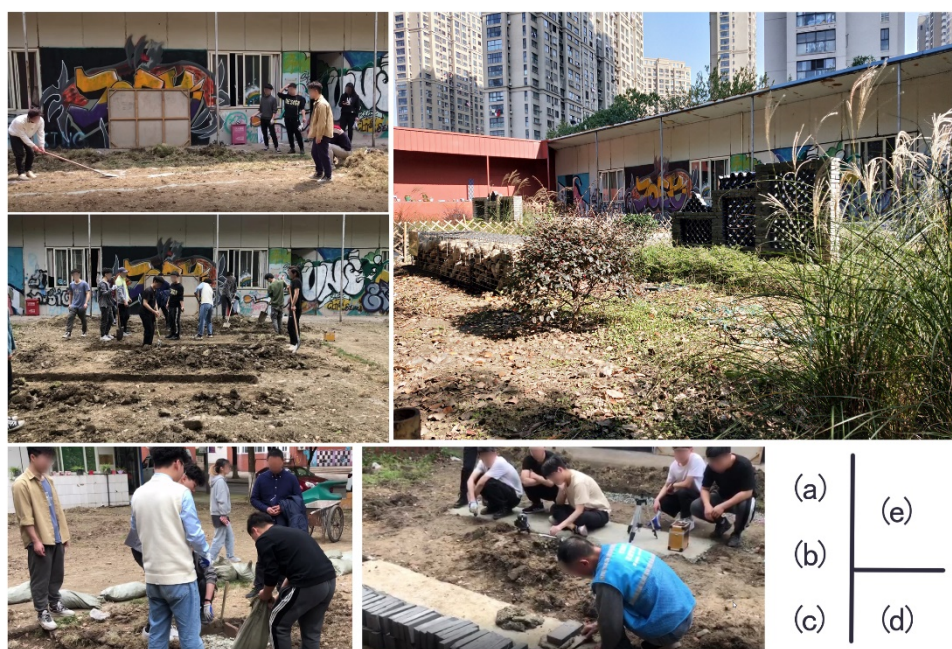
Figure 2. Garden construction scenes: (a) setting the design on the site; (b) digging the foundation of walls; (c) filling concrete in the foundation; (d) learning bricklaying from external tutors; (e) the completed garden. To conserve energy and protect the environment, students used local materials such as stones, plants, bricks and organic mulch, which were easy to procure, transport and maintain. (Images are reproduced with the permission from Xinqian Liu, a student of the experimental group who took these photos.)
