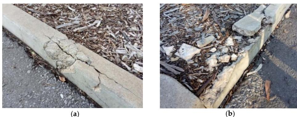
**Figure 2.** Failure of a kerb due to insufficient clear cover for reinforcement (a) Longitudinal crack after initiation, and (b) after failure.
