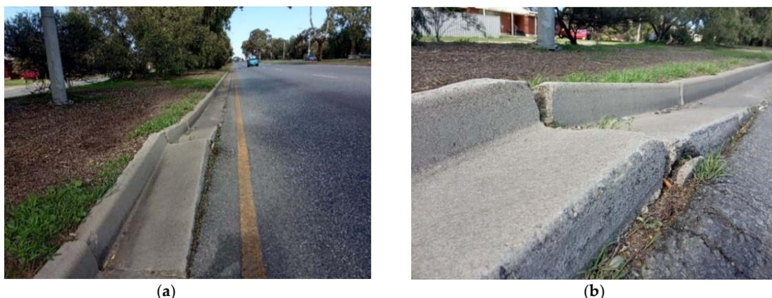
**Figure 3.** Upward displacement of a kerb due to expansive soil movement (a) view along the length, and (b) side view.
