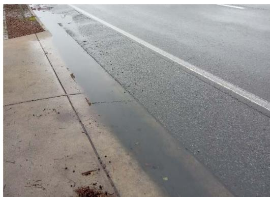
**Figure 5.** Faulty drainage due to differential movements of a kerb at entry.
