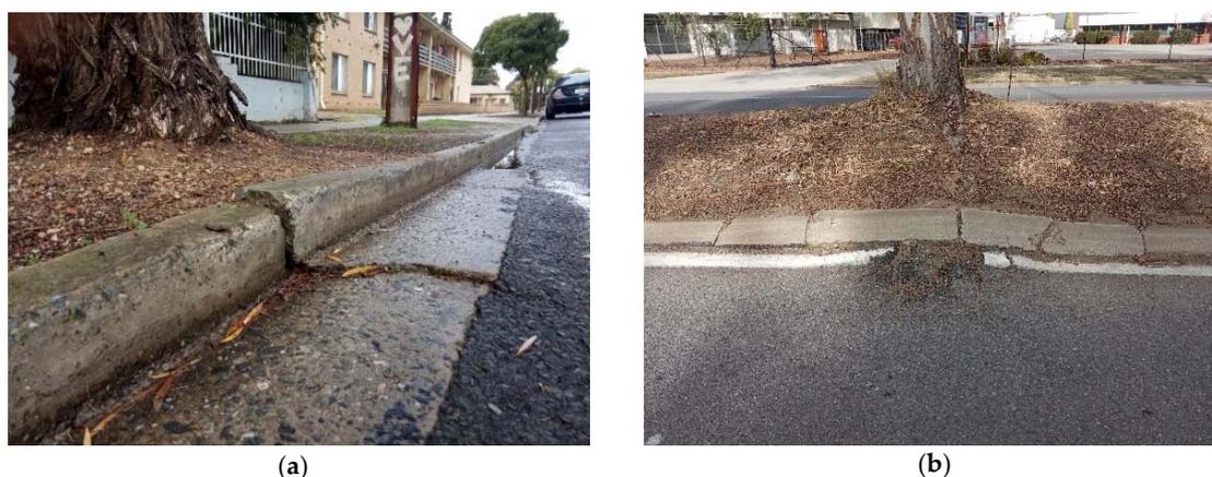
**Figure 4.** Damage to kerb caused by tree roots (a) single point breakage, and (b) multiple point breakage.
