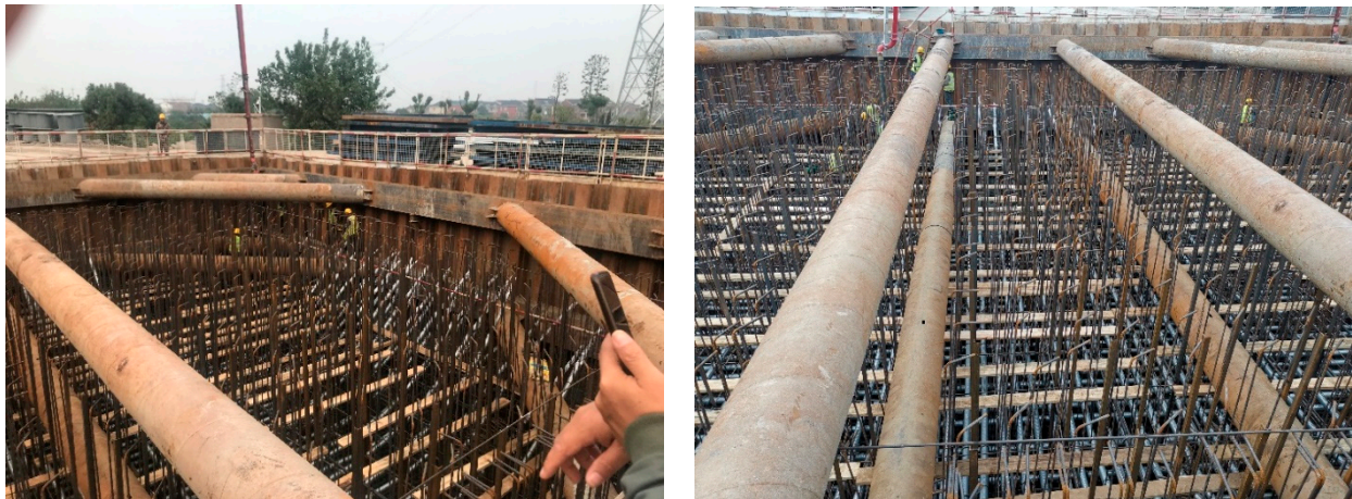
Figure 2. Layout of the pit support structure.
