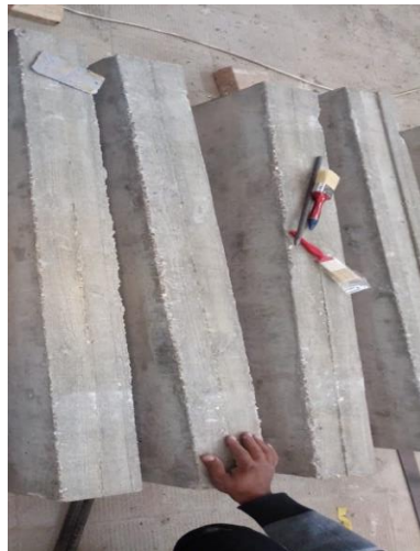
(b) Preparing the beam surfaces
