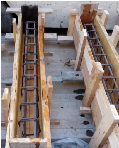
(a) Formwork and steel rebars
