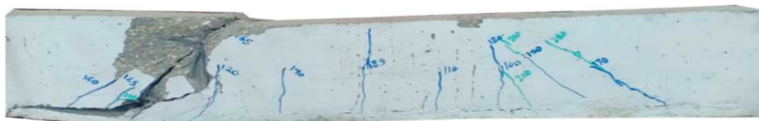
(g) Shear failure and end peeling of a beam (B7)
