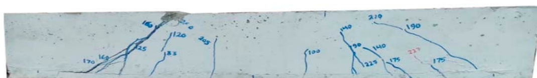
(e) Shear failure of a beam (B5)
