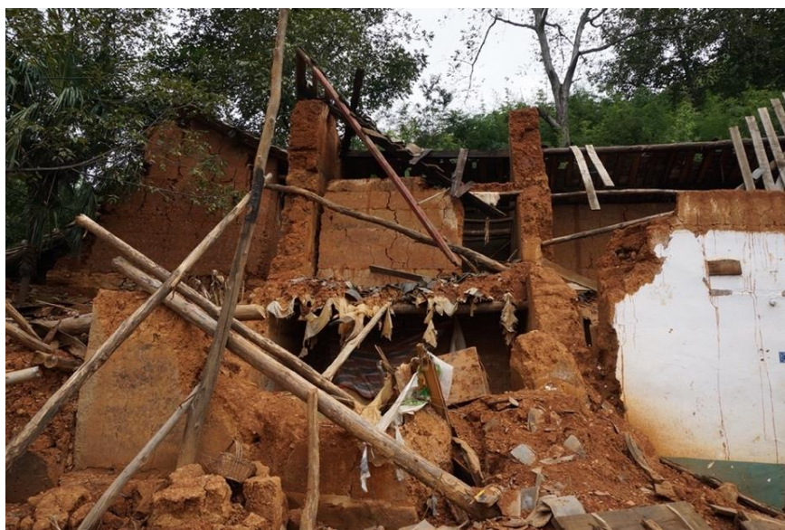
Figure 2. An old rammed earth house in Southwest China damaged after an earthquake.
