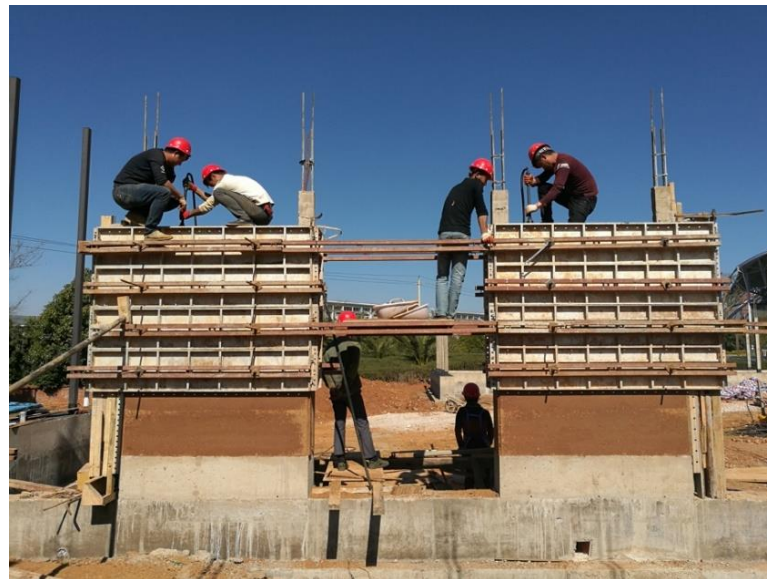
Figure 11. Rammed earth wall construction of the Terra Centre.
