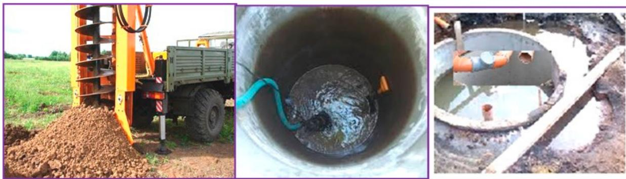
**Figure 6.** Drilling and installation work of the asbestos-cement casing pipe and equipment of the stop valves with a system of float valves on the pipe top. Photo taken by V. Kulagin and A. Ismagulova, 2018.
