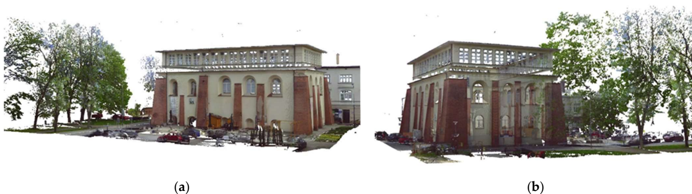
Figure 9. Current synagogue elevations obtained by scanning: (a) the south-eastern elevation; (b) the northwestern elevation.
