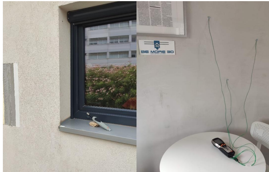
Figure 4. Thermal transmittance measurement process.
