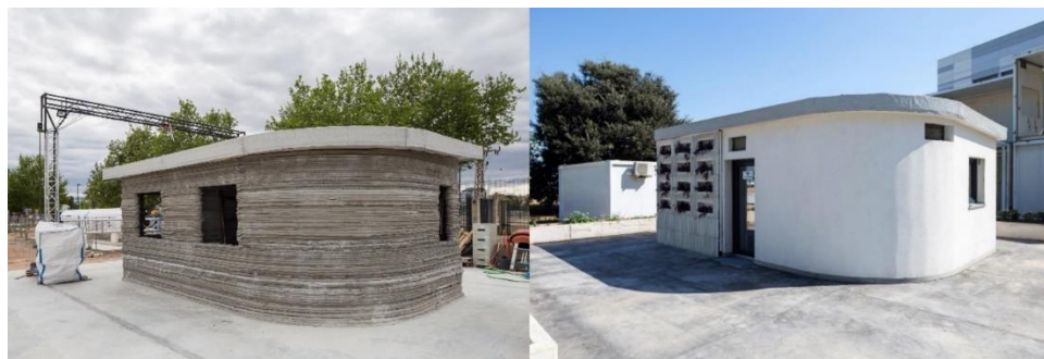
Figure 1. First 3D-printed house in Spain (raw and finished).
