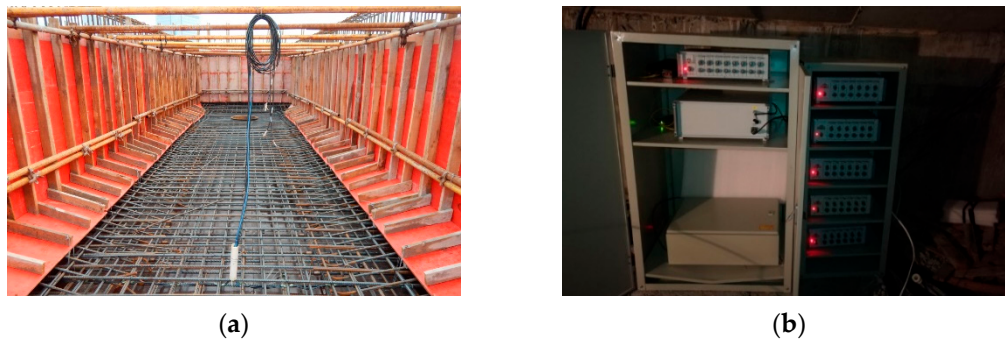
Figure 3. Field installation of the SHM system: (a) pre-embedded strain and temperature sensors; (b) data acquisition instrument.
