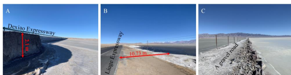
Figure 7. Status of expressway and road around Xiao Qaidam Lake (Photos (A–C) are corresponding to site 1/2/3 in Figure 1, respectively).
