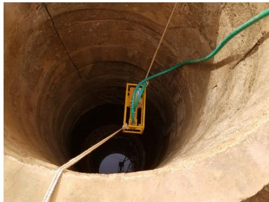
**Figure 4.** Surface solar pump riskily lowered into a well to pump the deep aquifer in Ramitenga.
