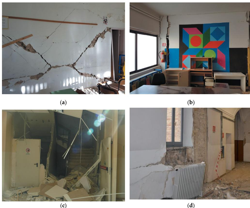
**Figure 1.** Damage to school buildings after 2009 L’Aquila earthquake: (a) diagonal and (b) vertical cracks in masonry infill panels; (c) collapse of internal partitions and damage to stairs; (d) damage to non-structural and heater elements (Di Ludovico et al. [7]).
