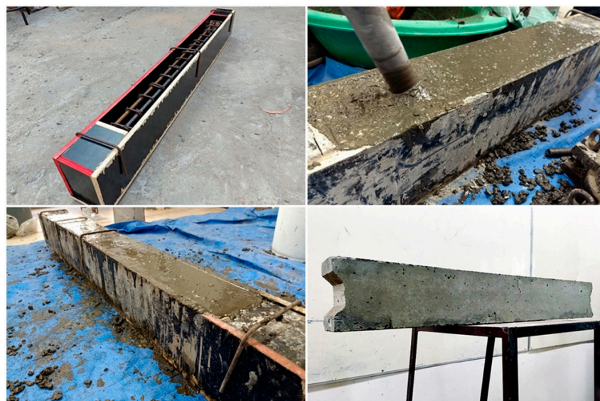
Figure 4. The beam casting process.
