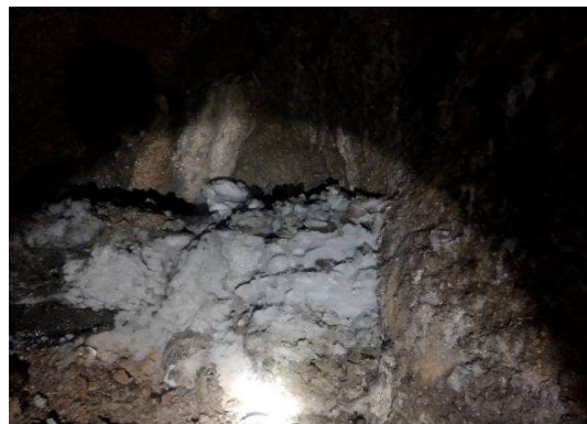
Figure 10. Solidifying effect of phosphoric acid and sodium silicate slurries.
