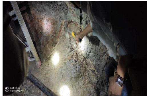
Figure 3. Sanding dolomite layer of Xiaopu 2# construction adit.
