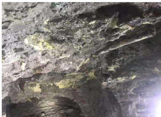
Figure 11. Effect after Malisan grouting.
