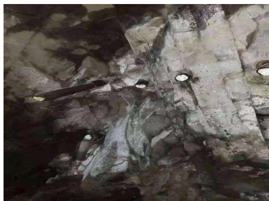
Figure 12. Effect after urea formaldehyde resin grouting.
