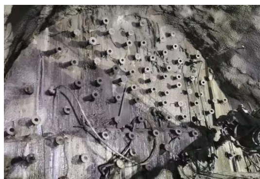
Figure 8. Actual layout of advanced grouting holes in the tunnel face.
