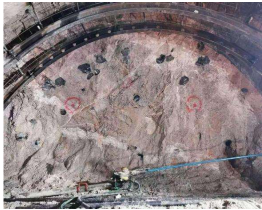
Figure 9. Grouting effect of upper-step excavation face.
