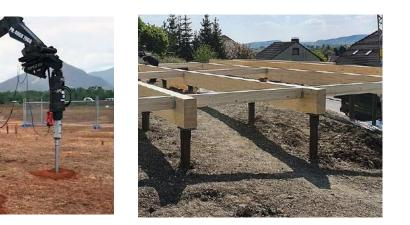
**Figure 4.** Mini-excavator and mini-shovel equipped with a hydraulic drill for the installation of foundations on poles by screwing.
