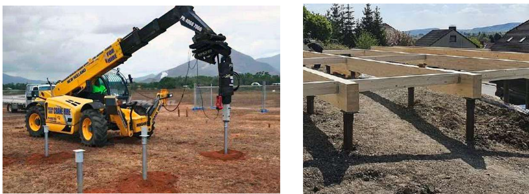
Figure 4. Mini-excavator and mini-shovel equipped with a hydraulic drill for the installation of foundations on poles by screwing.
