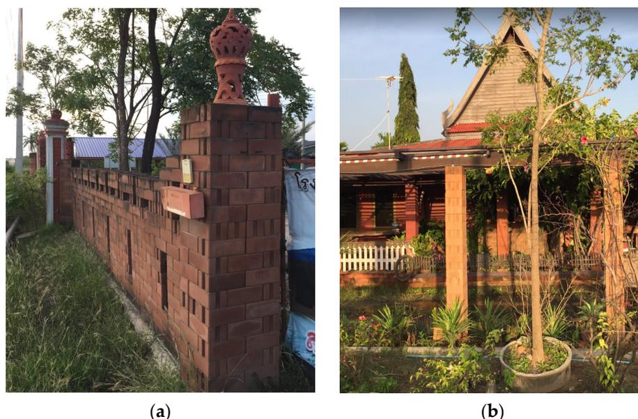
**Figure 1.** Use of cement clay interlocking bricks at Chachoengsao Province, Thailand (a) boundary wall, (b) walls and columns.
