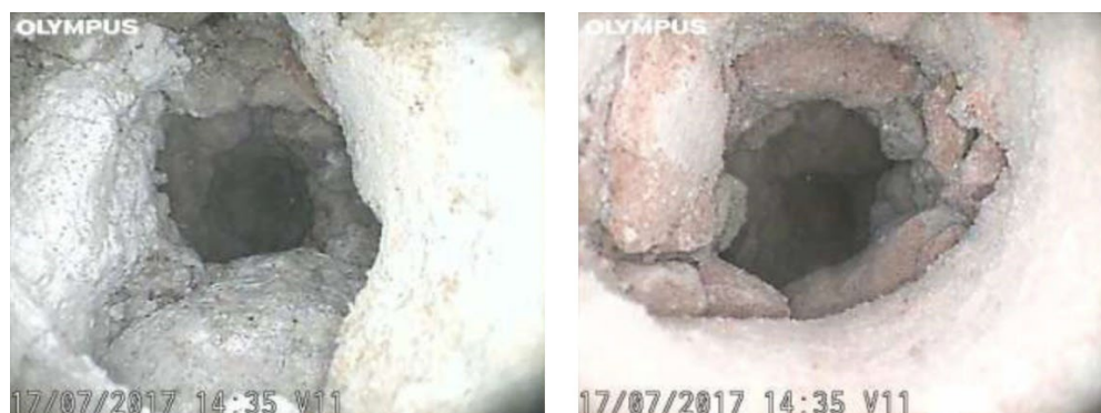
Figure 8. Extract of in situ investigations [21]. In particular, photographs of videoendoscopy V11—from intrados. On the left, view at 15 cm from the start of the drill, filling in unbound material; on the right, image at 10 cm from the start revealing of the drill, brick and mortar elements.
