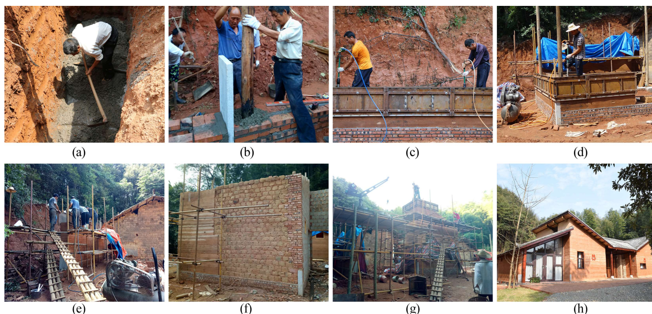
Figure 15. The construction process of renovated dwellings. (a) Foundation construction. (b) Column-in-wall construction. (c) Column-in-wall construction. (d) Wall corner construction. (e) Moulds installation. (f) The intersection of the new wall and the old one. (g) Wall construction. (h) Renovated dwellings.
