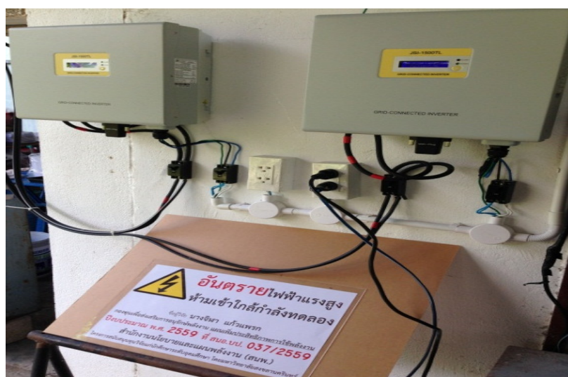
Figure 3. JFY® JSI-1500TL grid-tie inverter.
