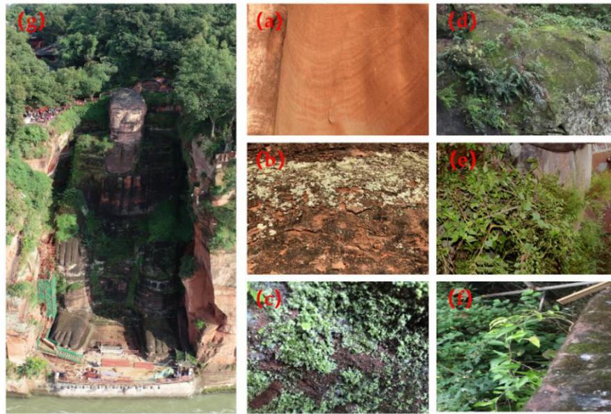
**Figure 1.** Body of Leshan Giant Buddha covered by different organisms. (a) naked rock; (b) surface of sandstone covered with lichens; (c) bryophytes-covered rock; (d) rock growing with fern; (e) rock growing with gramineous plant; (f) rock growing with shrub; (g) buddha body of Leshan Giant Buddha.
