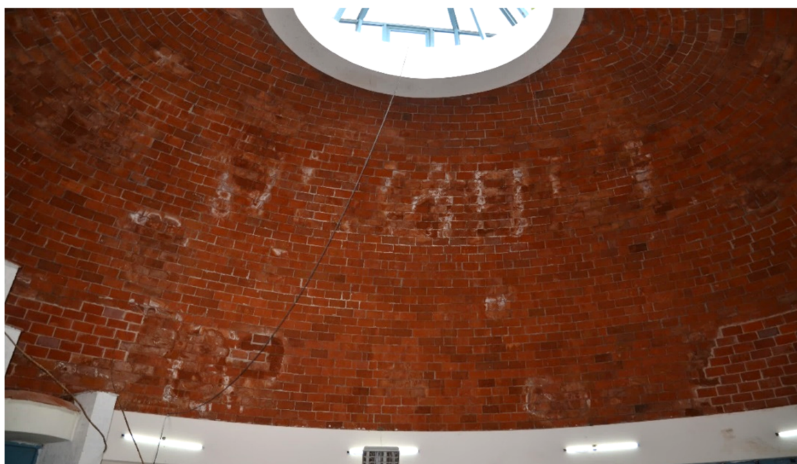
Figure 26. Efflorescence patterns at the intrados of the domed classrooms (photo by the authors).
