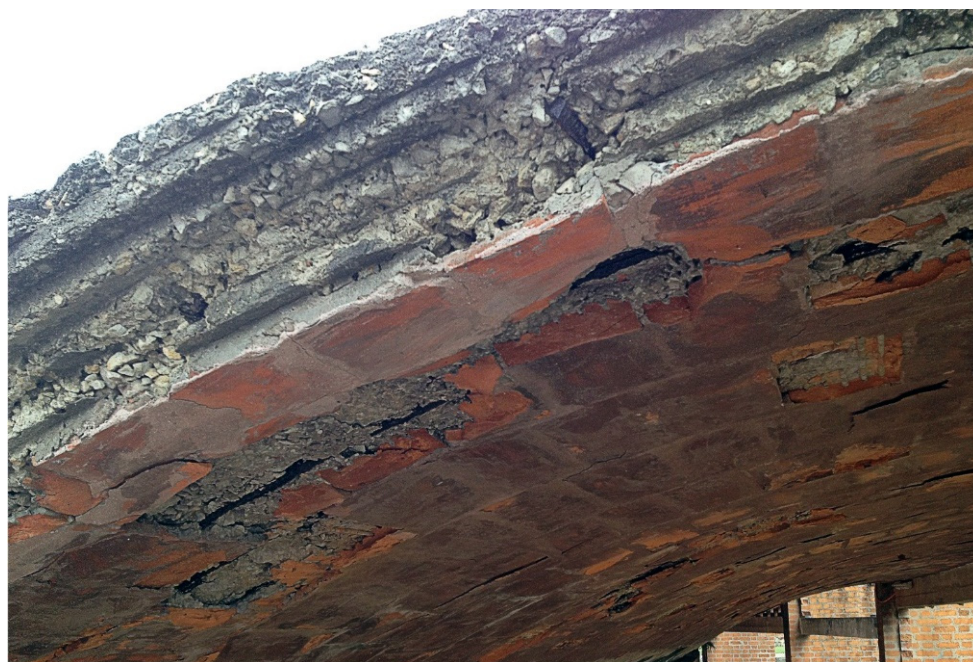
Figure 23. One of the vaults replaced with plain concrete vaults. The poor quality of the materials employed resulted in delamination and consequent exposure of steel rebar (photo by Luca Valisi).
