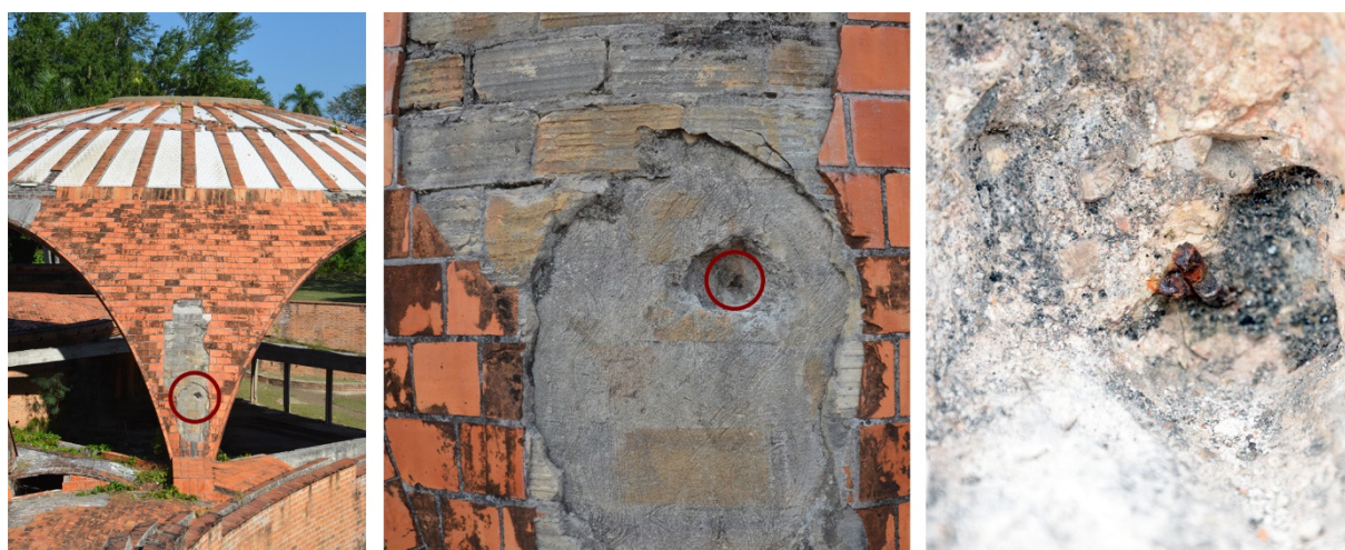
Figure 3. The pendentives of the dance pavilion's dome. The loss of the outermost layer of tiles unveiled the presence of reinforced concrete. The picture on the right shows the visible tie wire.
