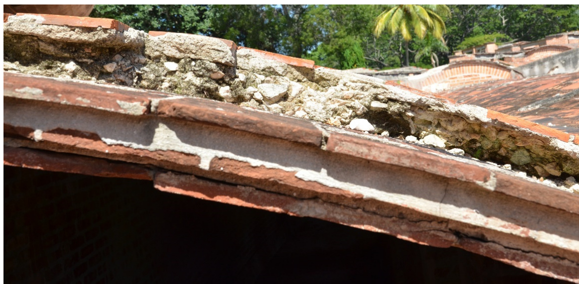
Figure 21. Current stratigraphy of the vault covering the lower corridor of the gusano building (photo by the authors).
