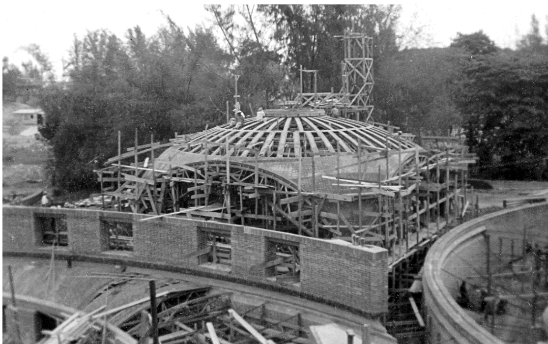
Figure 10. One of the dance pavilions after the concrete casting. The picture clearly shows the concrete framework hidden beneath the current clay tile covering (ISA archive).
