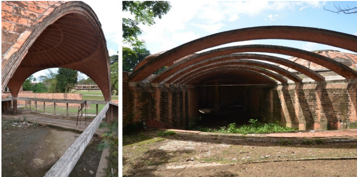
Figure 5. The deceptive appearance of the side finishing of the domes and vaults of the School of Ballet, displaying alternating layers of clay tiles and mortar (photo by the authors).
