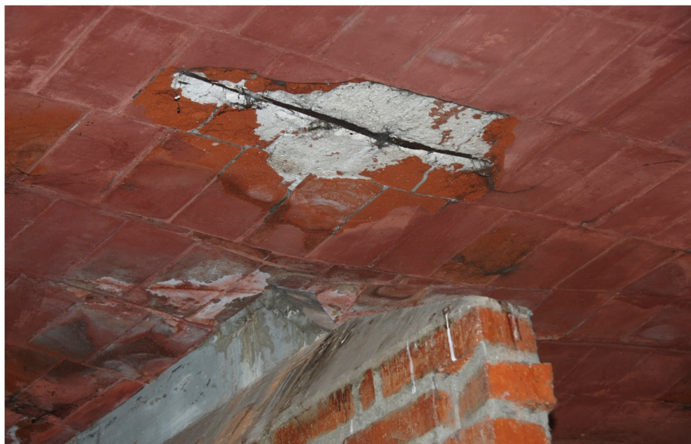
Figure 19. Exposed steel rebar at the intrados of the pasillo (photograph by the authors).
