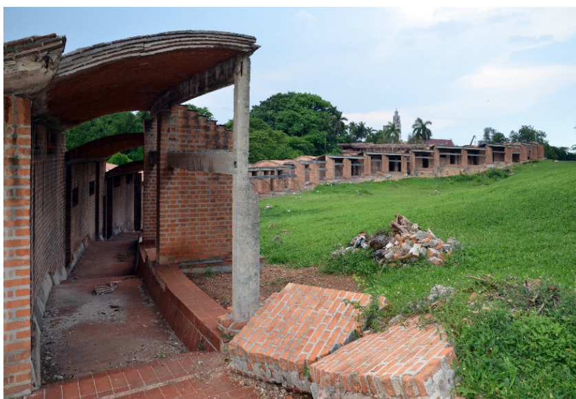
Figure 24. The cracks running along the crown of the vaults covering the upper corridor of the gusano building (photo by the authors).
