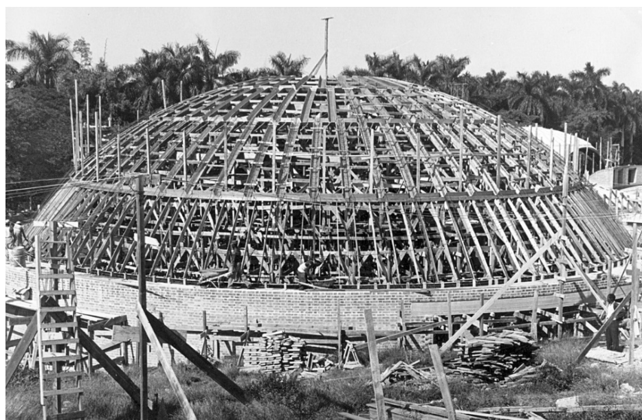
Figure 4. The School of Ballet's choreography theater during construction. The photograph depicts the wooden formworks for the casting of the dome's concrete ribs and rings (ISA archive).
