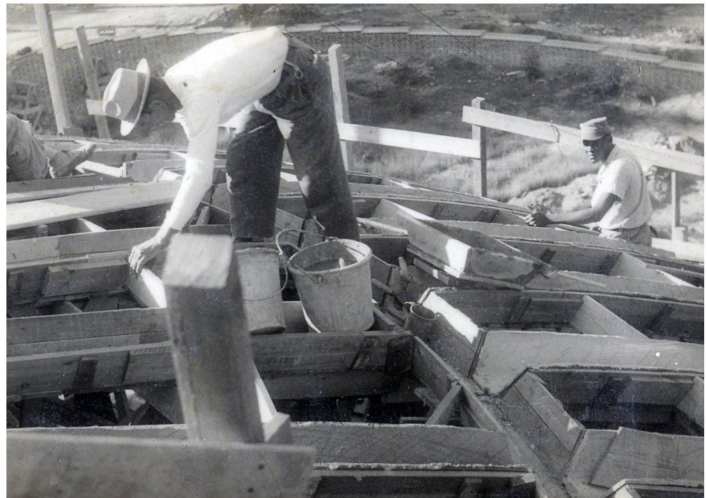
Figure 8. The wooden formworks of the ribs and rings of the choreography theater while being coated with clay tiles on the inside (ISA archive).
