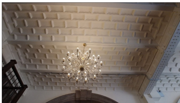
Figure 9. Original ground floor ceiling and steel structure retained and exposed at 30 James Street.
