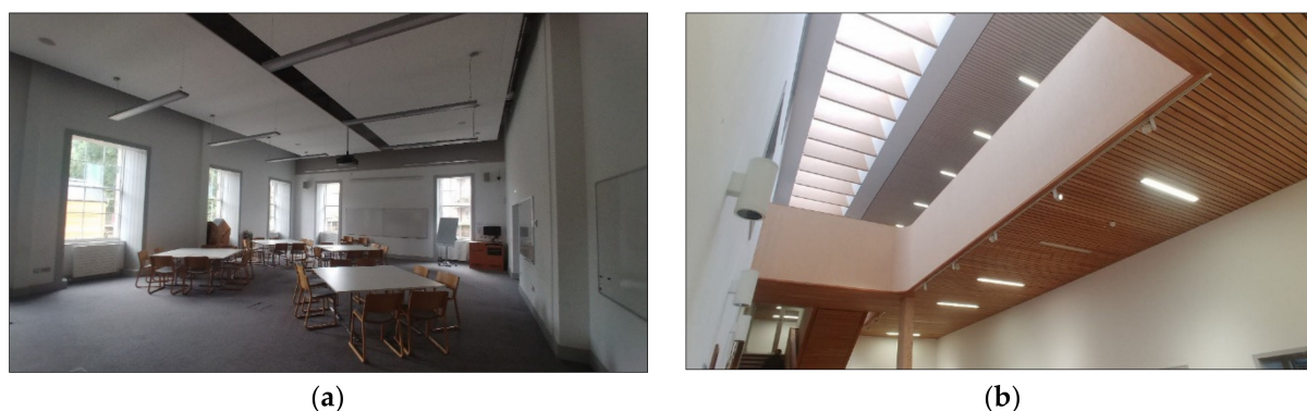
Figure 5. Passive design in the ECCI (a) Retained large sash windows from original structures providing daylighting and solar gains; (b) Diffused daylighting and electronically controlled opening vents in the ECCI central atrium; author's photographs.
