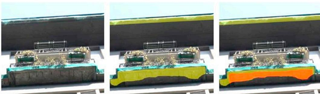
**Figure 5.** Corner's surfaces (in yellow) are affected by gaps, the remaining parts (in red) can be considered less dangerous as their falls will probably be stopped by lower balconies.
