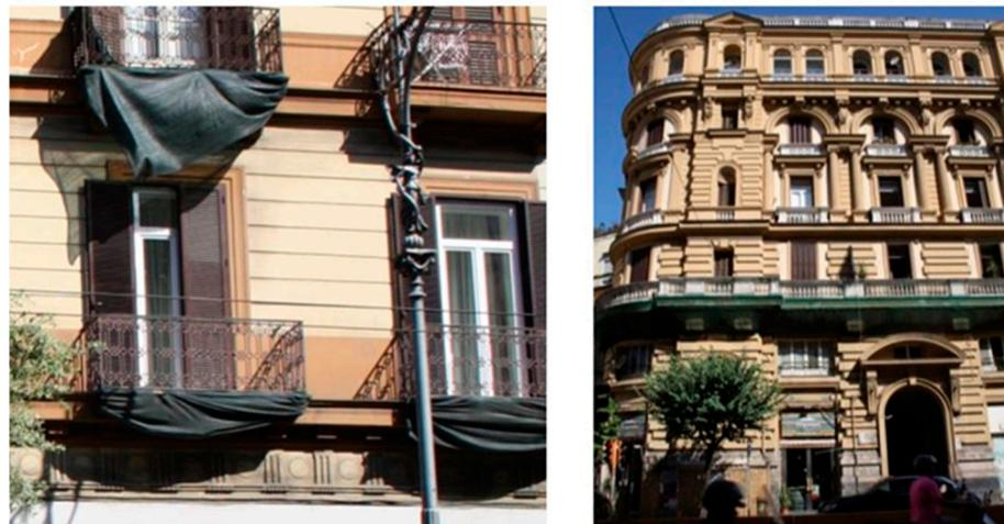
**Figure 3.** Examples of protective measures (balcony at the first floor and containment nets) along the examined avenue.
