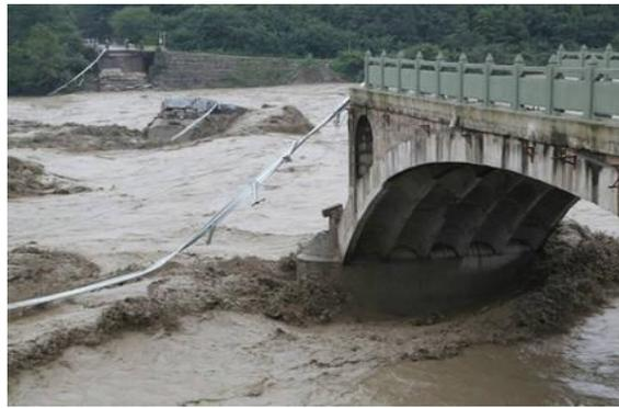
**Figure 1.** Collapsed Sichuan Panjiang Bridge [2].
