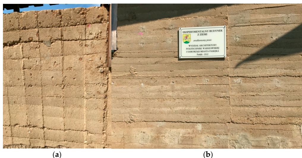
Figure 17. Texture of the external walls built with raw-earth technology (a) screen wall built from raw and straw blocks (b) external wall built as rammed earth in formwork. Photos taken during architectural and technical site visit on 1 August 2018.
