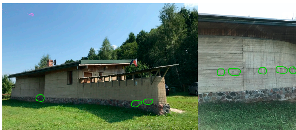
Figure 15. View on the north elevation with visible defects in the stone plinth zone and visible points after the tie bars were used during construction. Photos taken during architectural and technical site visit on 1 August 2018.
