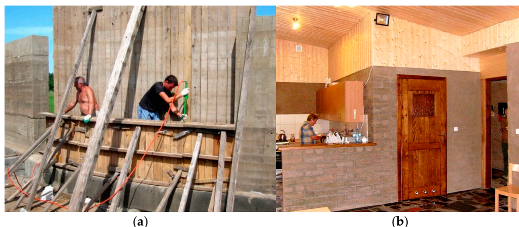
Figure 2. Building under construction and completed: (a) Compacting of raw earth mixture with pneumatic compactor in wooden formwork (b) Internal walls: pressed earth blocks with no finish (left side). Clay and straw compacted mass blocks finished with earth plaster (right side of door) and with natural finish (right side).
