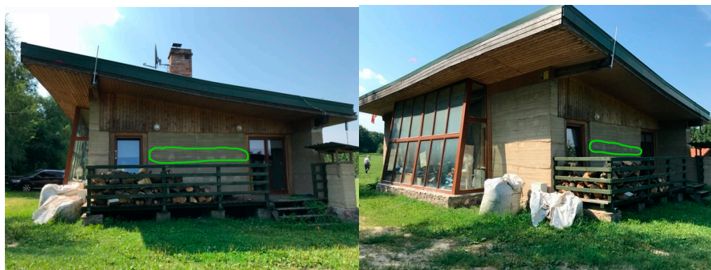
Figure 13. View on the eastern elevation with visible points after tie were bars used during wall construction. Photos taken during architectural and technical site visit on 1 August 2018.
