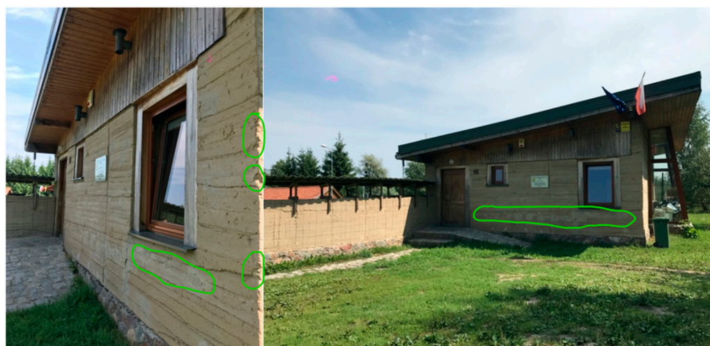
Figure 12. View on the western elevation with visible points after tie bars were used during wall construction and defects in the corner of the wall. Photos taken during architectural and technical site visit on 1 August 2018.
