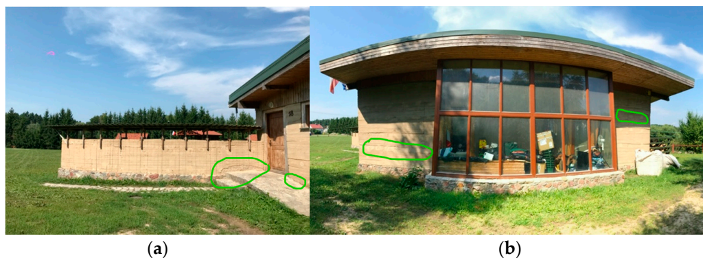
Figure 14. View on the south elevation (a) with visible defects on the screen wall in the plinth zone near landing and flight of stairs. (b) On south elevation points after tie bars were used during wall construction are visible near veranda. Photos taken during architectural and technical site visit on 1 August 2018.
