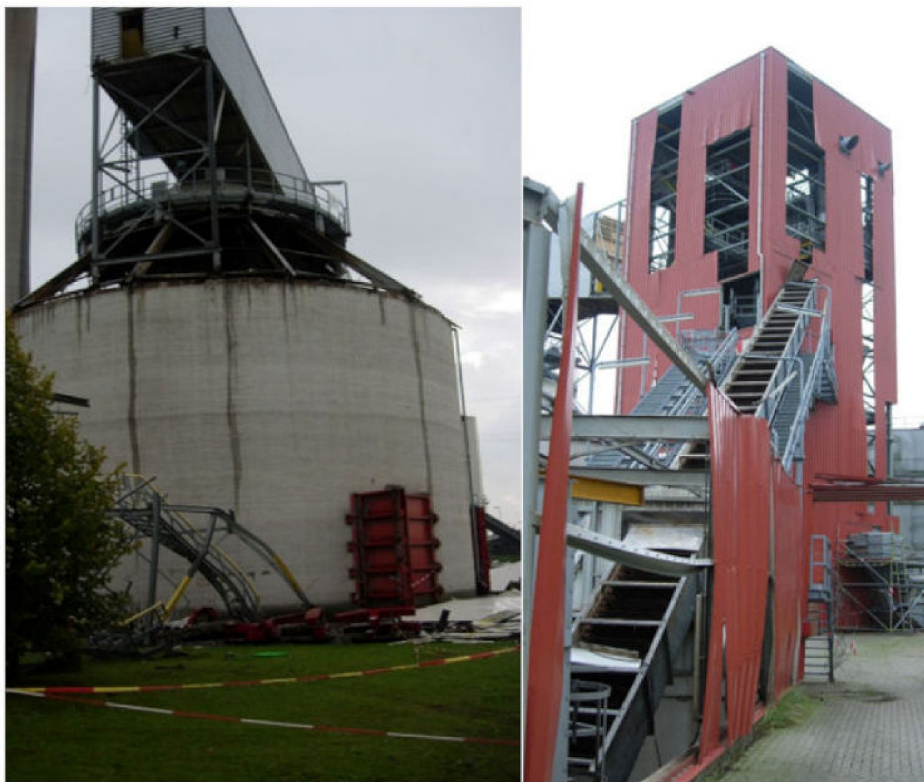
Figure 4. Damage following RDF Fire and Explosion (photo—J. Januszewski).
