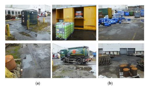
**Figure 10.** Case study B—multiple sources of diffuse pollution: (**a**) oil storage area with interceptor drain; middle: chemicals storage area and example contractor vehicle on site; (**b**) drum and skips storage area (above) and contaminated surfaces at the eastern side of the factory (below).
