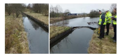
Figure 13. Inlet channel to the primary pond and oil boom at discharge into that pond.
